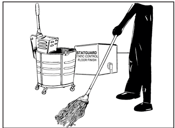
Figure 4. Applying floor finish.
